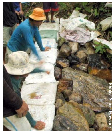
Constructing a check dam to collect rainwater in Koh Lanta, Thailand.
